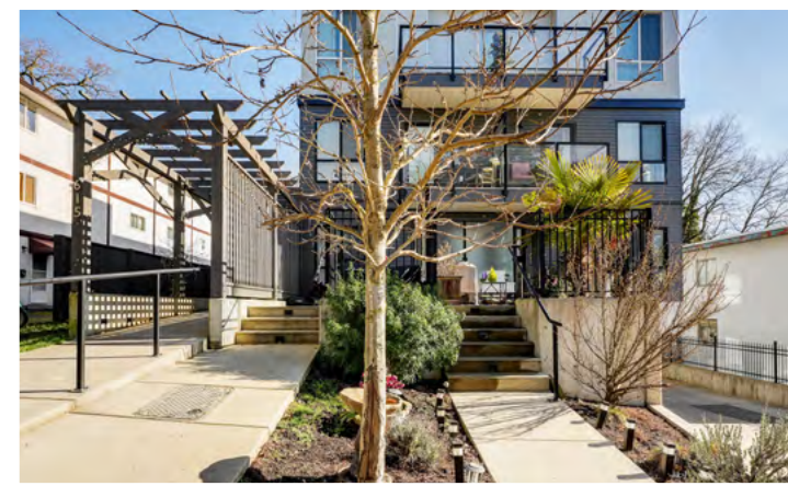
FRONT OF BUILDING
