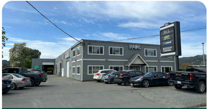
FRONT OF BUILDING
