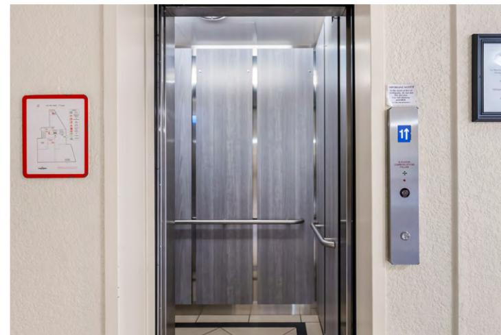
COMMON AREA - ELEVATOR
