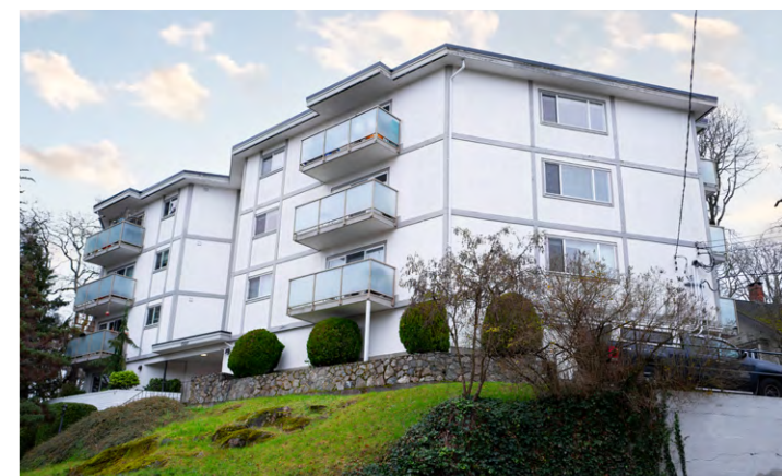
WEST SIDE OF BUILDING
