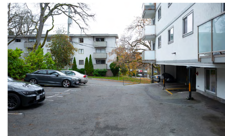
BACK OF BUILDING / PARKING
