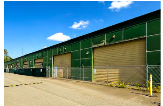
WAREHOUSE LOADING DOORS
