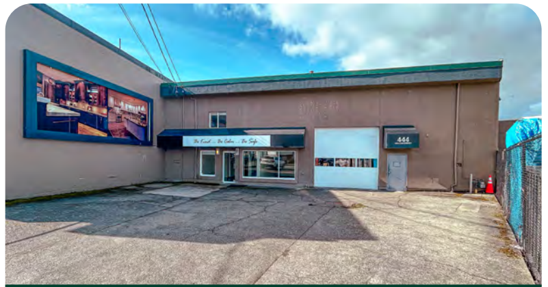
FRONT OF BUILDING
