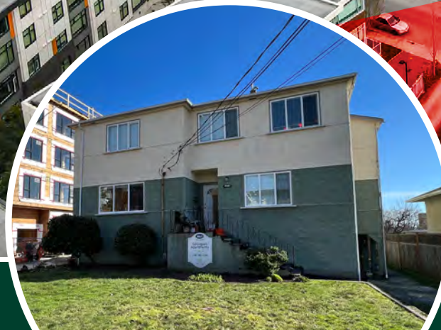
The Georgian Apartments
